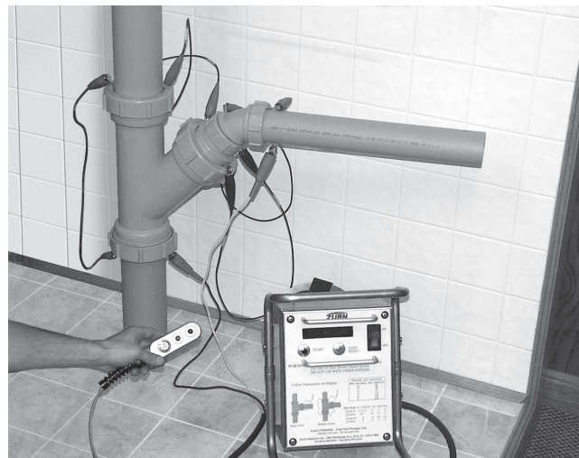
Figure 2-13 Fusion Lock Process in Operation
